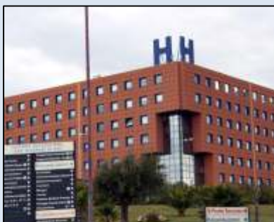
CONSTRUCTION AND RESTORATION OF CIVIL AND INDUSTRIAL BUILDINGS
